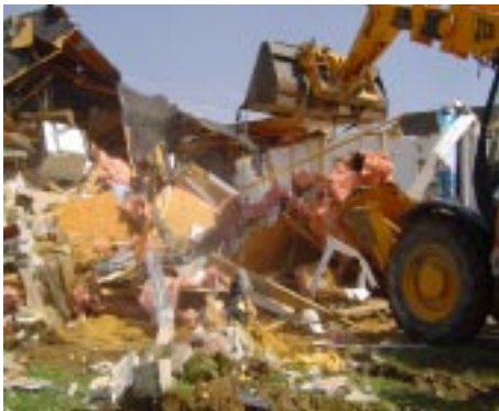
Bulldozer moves debris
