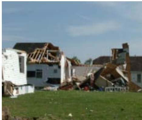
Tornado cuts swath through Navy family's house
