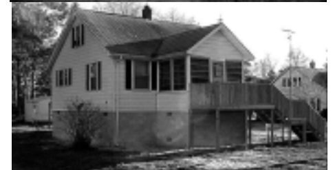
Before and After Pictures of a Home Elevation in Accomack Photos courtesy of David Fluhart.
