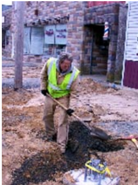
Streetscape improvements underway in downtown Exmore
