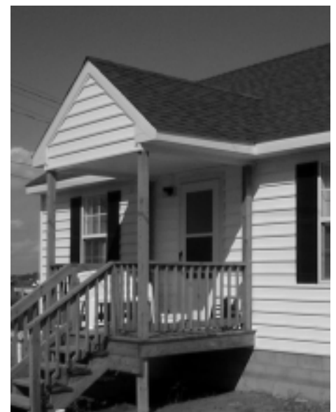
One of 6 new flood code compliant homes on Tangier Island
